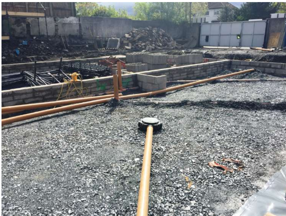
Photo 12 – Radon sump
