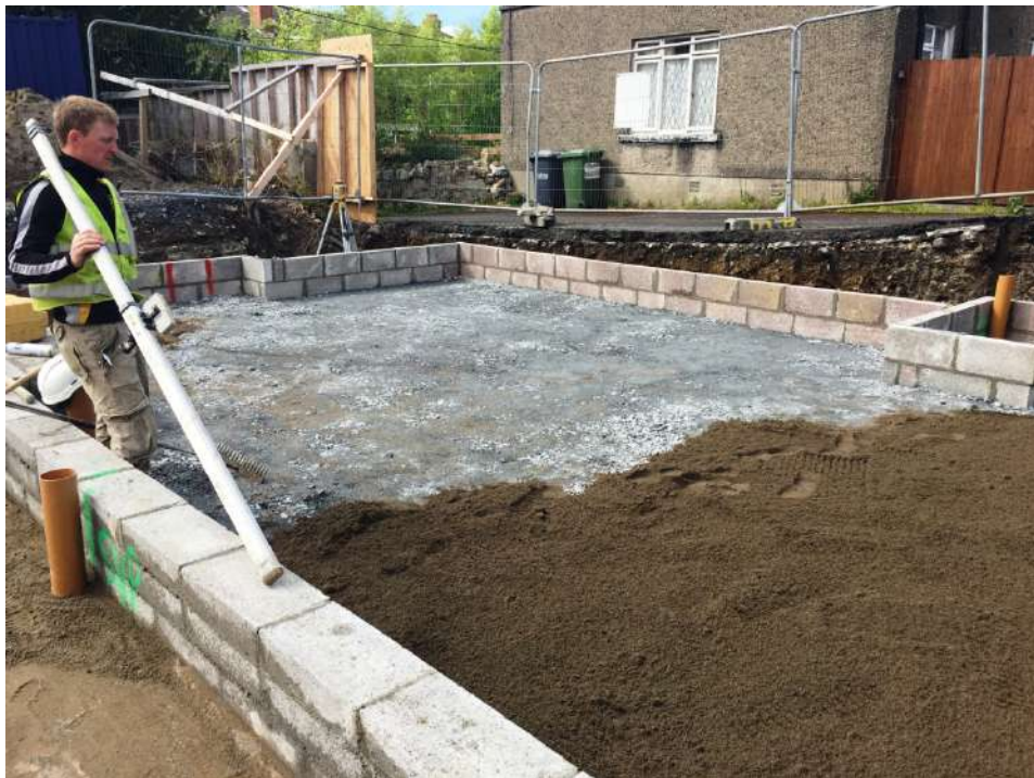
Photo 8 - Sand blinding in preparation for Radon Barrier / DPM
