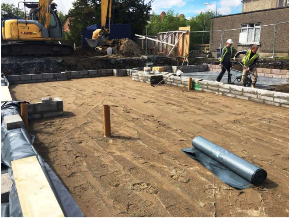
Photo 5 – Sand blinding in preparation for Radon Barrier / DPM
