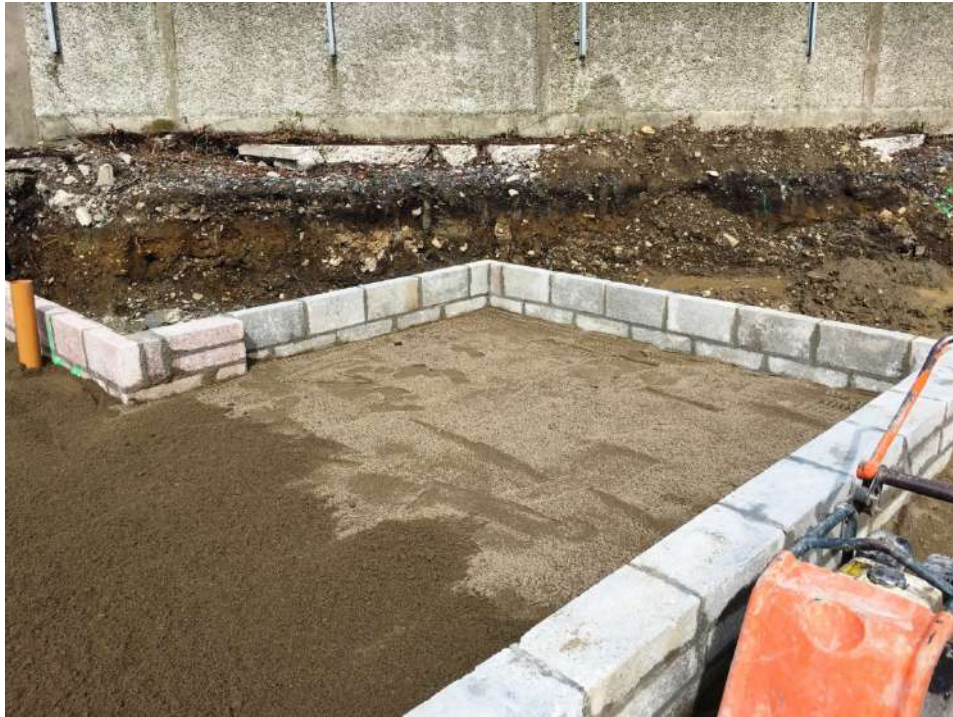
Photo 9 - Sand blinding in preparation for Radon Barrier / DPM
