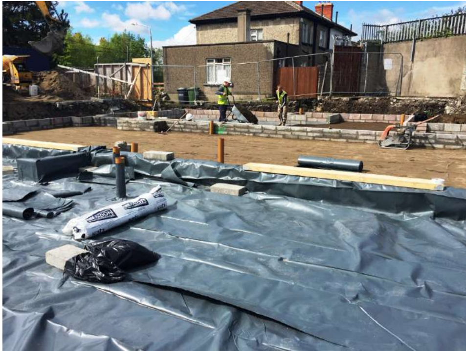
Photo 7 – Radon Barrier and DPM being laid out
