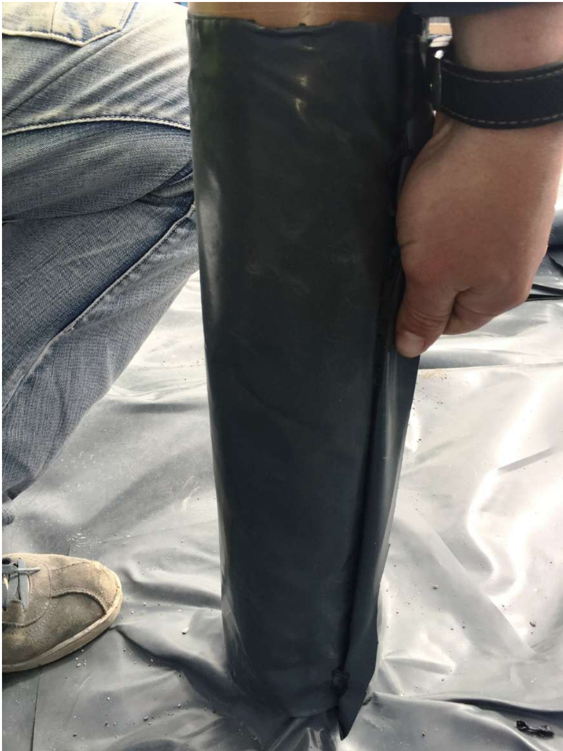
Photo 6 – Drainage pipe with DPM/Radon wrap
