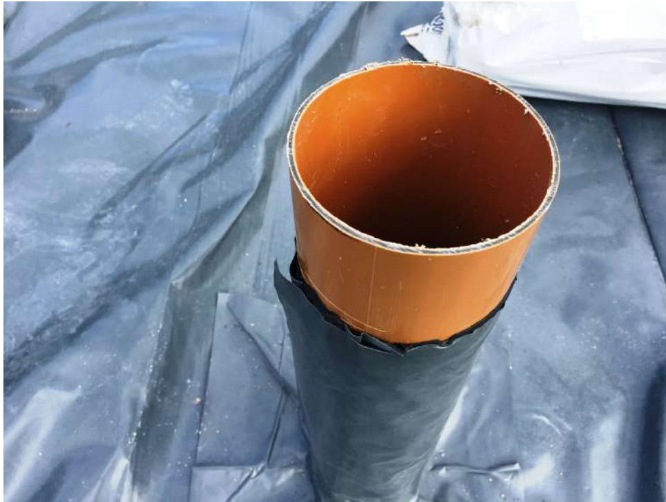
Photo 11 – Waste Pipe with Radon/DPM wrap
