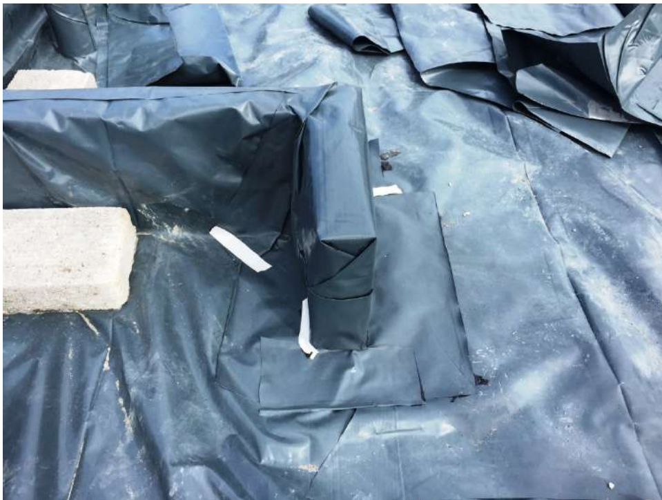
Photo 10 - Corner detail being formed
