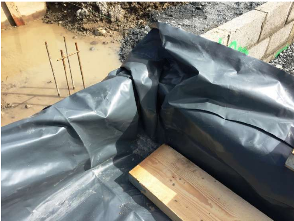
Photo 4 – Corner detail being formed
