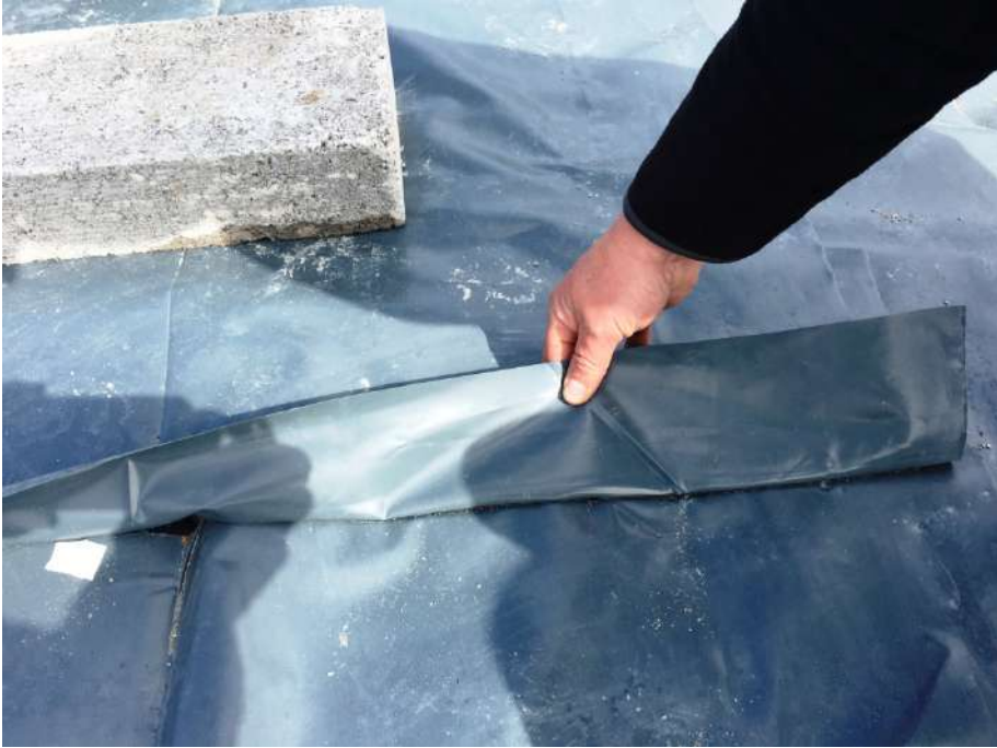
Photo 3 – Inspection of lapped and tapped joints
